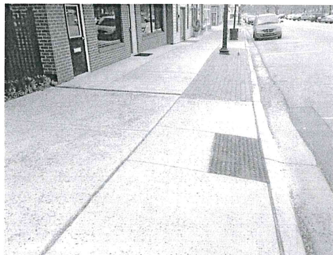
Wheelchair curb ramp on Main Street
