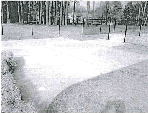
North Garner Dog Park handicap spaces under construction, April 2015
