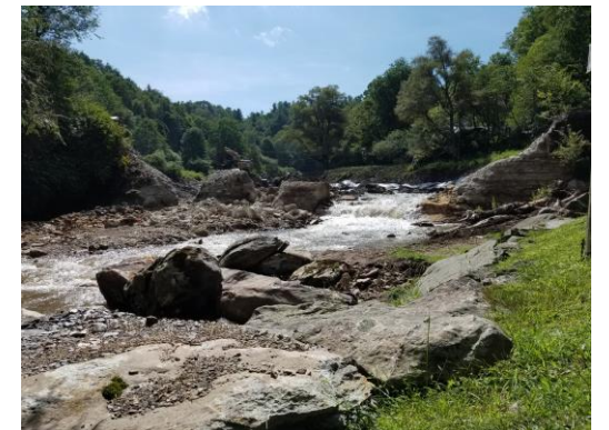
Pictures from Payne Branch Dam Removal
